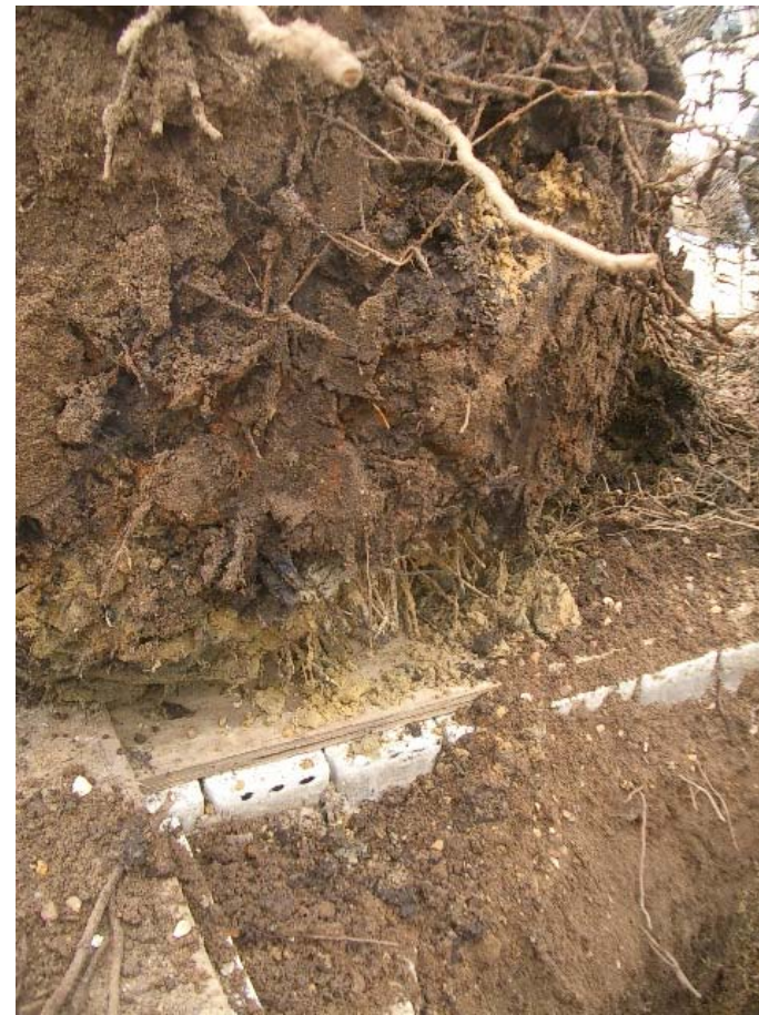
Tree 2 discoloration indicating some water logging of root-ball base
