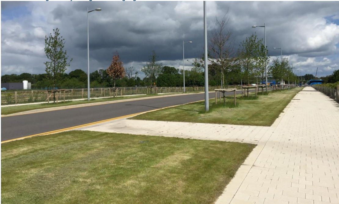
Plate 3 1: Existing Footway arrangement along High Cross
