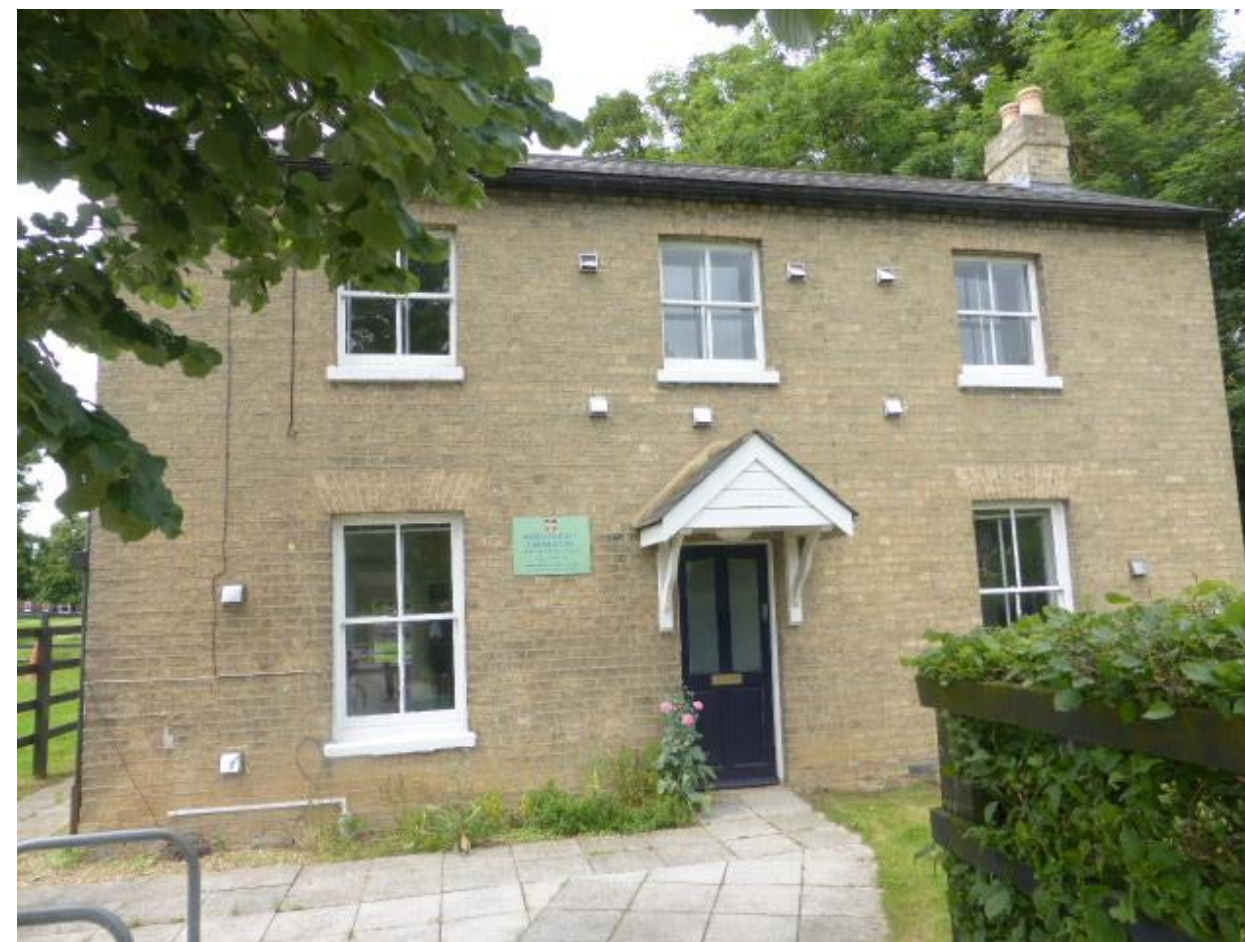
Figure 4.12 Merton Hall Farmhouse, principal east façade. Note the additions of vents, detracting from the quality of the façade
