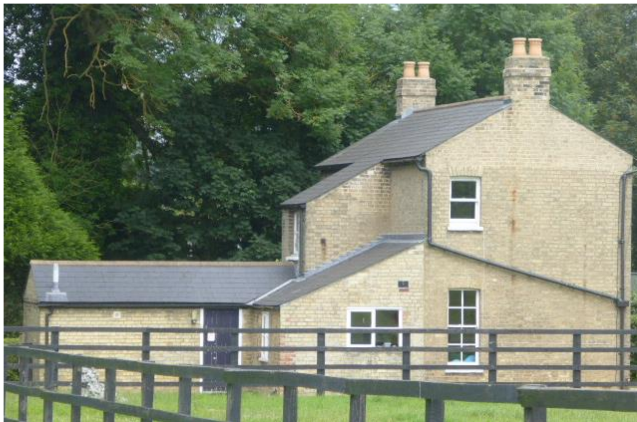
Figure 4.13 Merton Hall Farmhouse from the south west. Note the brickwork showing additions to the rear of the original building
