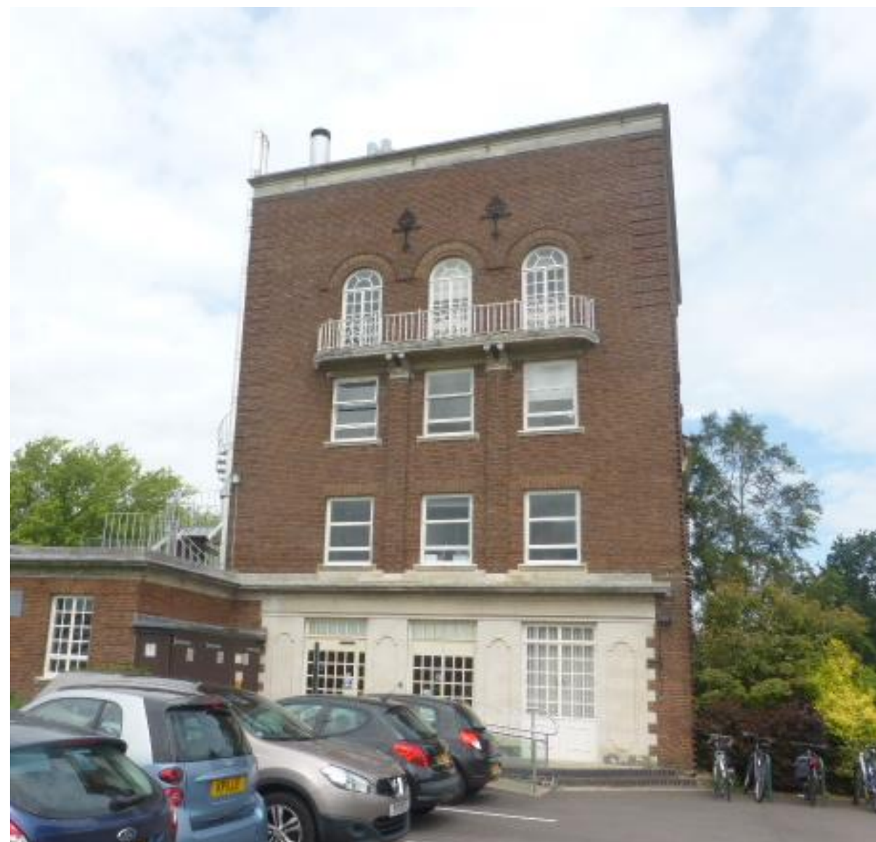
Figure 4.4 Vet School Teaching Block, southern section south façade
