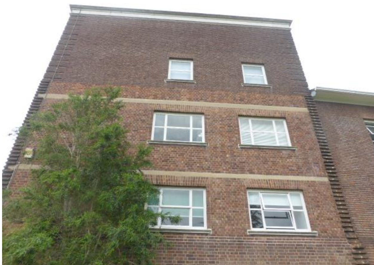
Figure 4.3 Vet School Teaching Block, southern section east façade. Note the poor quality staggered brickwork, which detracts from the façade
