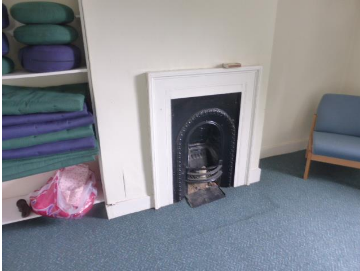
Figure 4.15 Merton Hall Farmhouse, first floor front room (north), showing register grate fireplace
