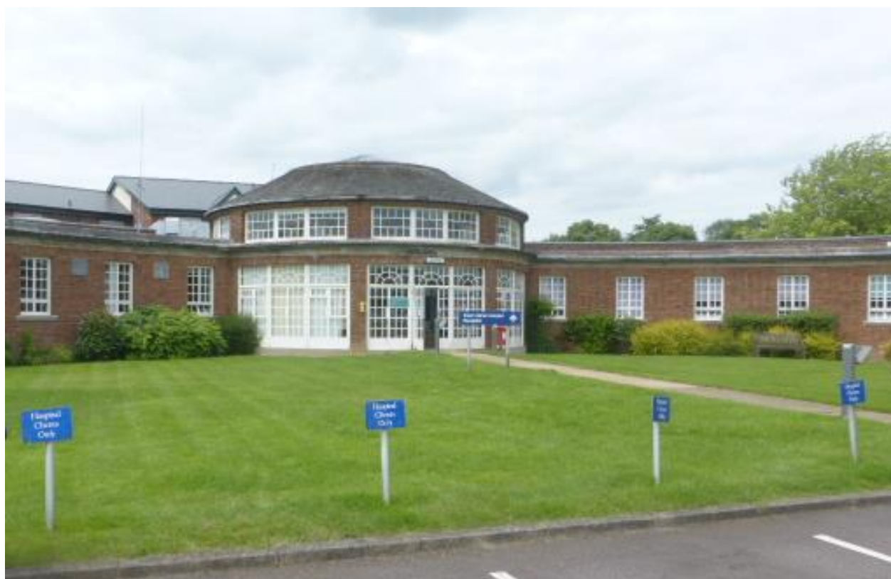
Figure 4.5 Vet School Hospital Block, principal east façade
