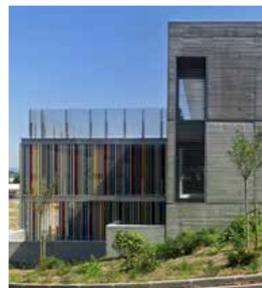
22. Parking structure in La Coruna: vertical variation in materials and variation in massing by treating the core separately
