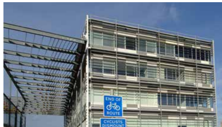
17. Rooftop Plant - minimal - impacts can be minimised by setting back from frontage line
