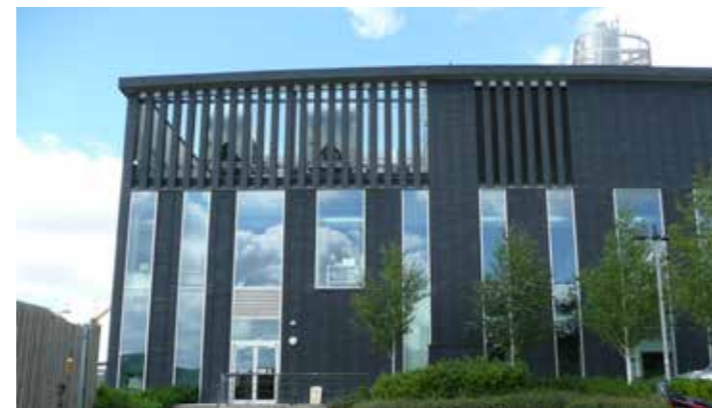
18. Rooftop Plant - medium plant integrated within the elevation of the building
