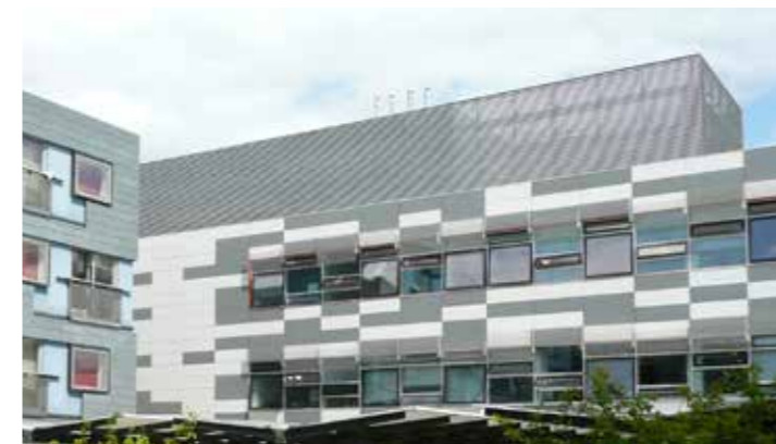
19. Rooftop Plant - screening of a large amount of rooftop plant space
