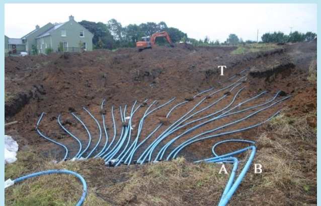
Figure 9: Image showing installation of surface collector loops for a ground source heat pump system prior to being covered and landscaped.
