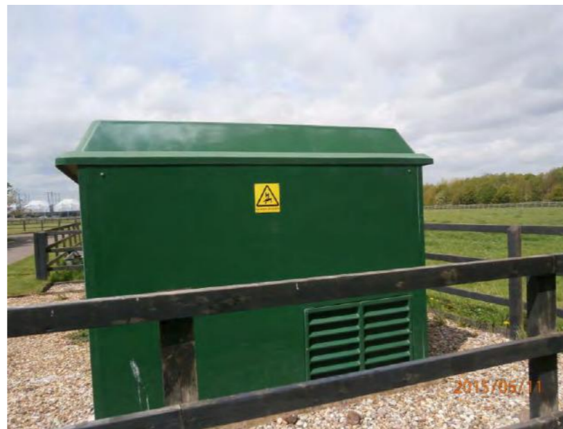
PHOTO 41 - Electrical Infrastructure north of School of Veterinary Medicine
