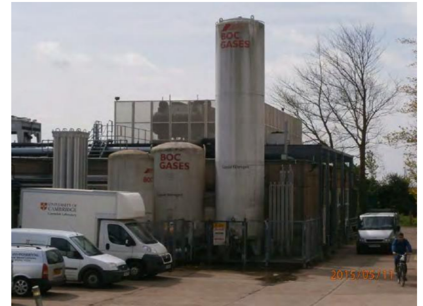
PHOTO 27 - Liquid nitrogen tanks adjacent to Cavendish Laboratory
