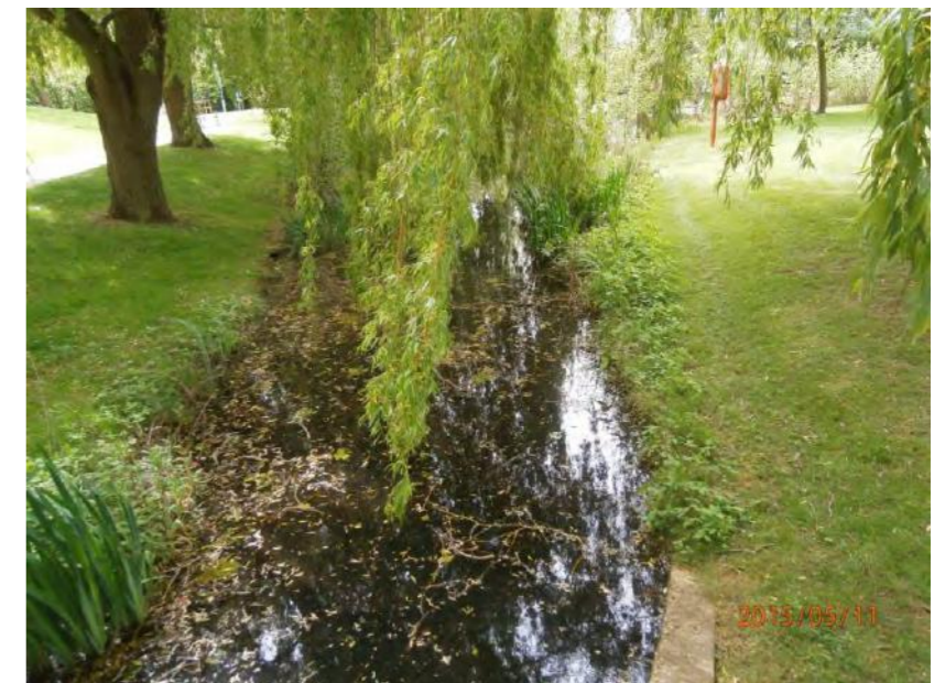
PHOTO 48 - Drainage channel to the south of Cavendish Laboratory
