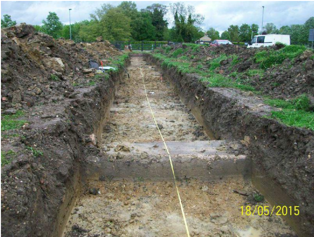
TR22 – Buried brickwork of former outbuildings south of Merton Hall Farm
