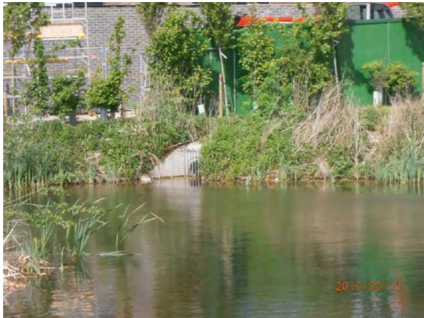
PHOTO 22 - Pond behind Institute for Manufacturing showing drainage structure.
