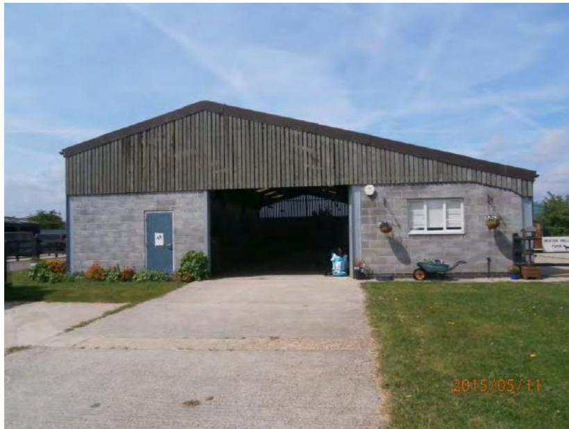
PHOTO 37 - Barn storage part of School of Veterinary Medicine
