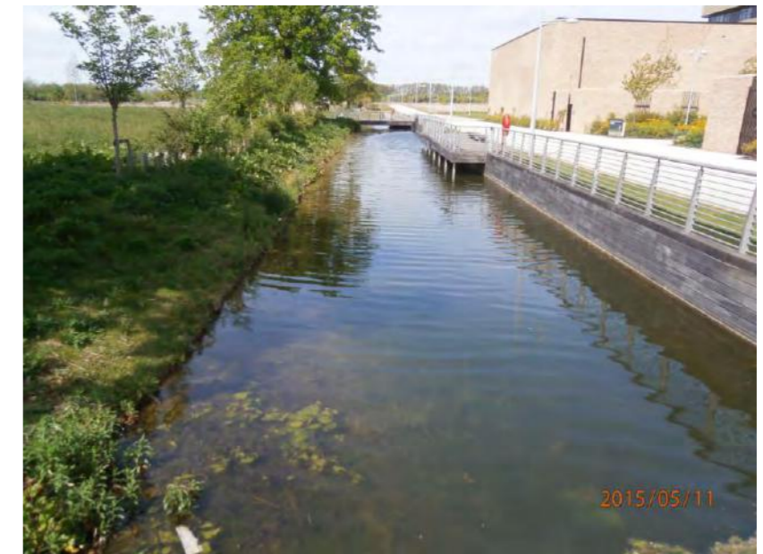
PHOTO 18 - Canal looking west south of Materials Science building
