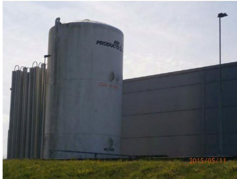
PHOTO 13 - Schlumberger liquid nitrogen tank located north of laboratory.
