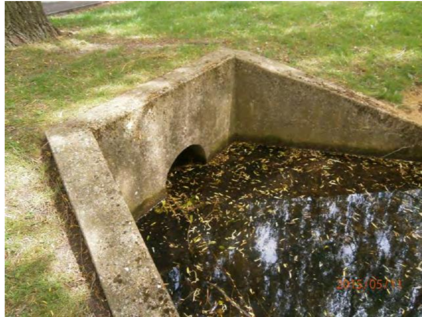
PHOTO 49 - Drainage channel to the south of Cavendish Laboratory
