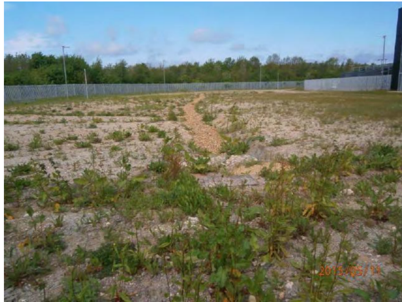
PHOTO 7 - Area west of Former Phase 2 Shorts Site, showing gravel filled drain.
