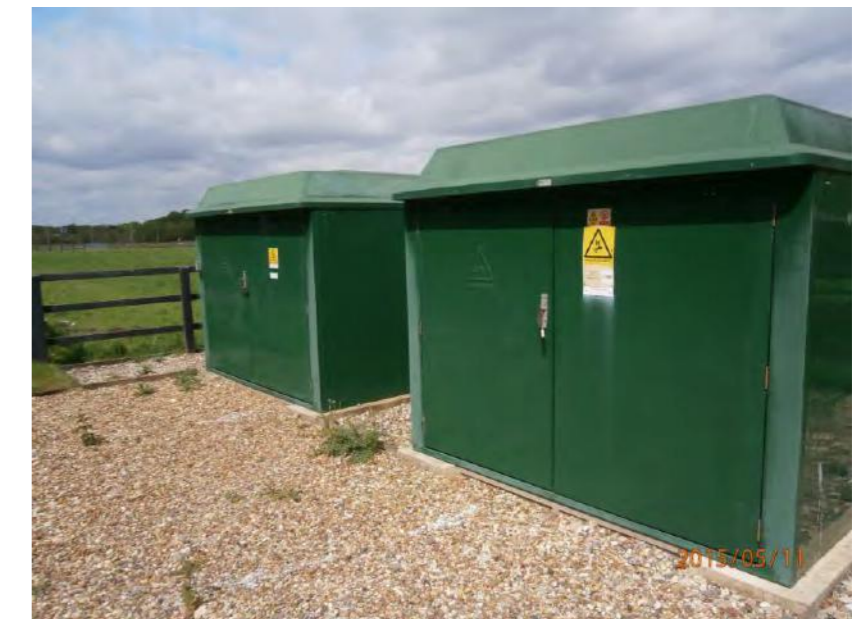
PHOTO 42 - Electrical Infrastructure north of School of Veterinary Medicine
