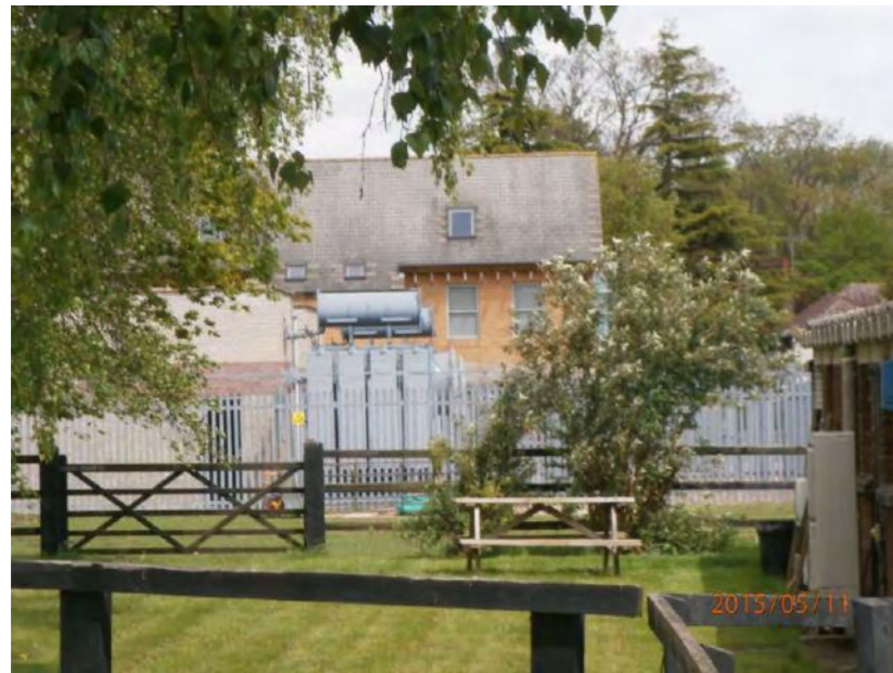
PHOTO 43 - Electrical Substation (in distance of) off Madingley Road on northern site boundary looking north.
