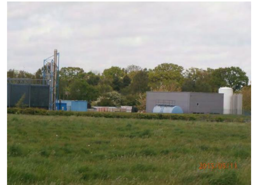
PHOTO 45 - Schlumberger tank storage area
