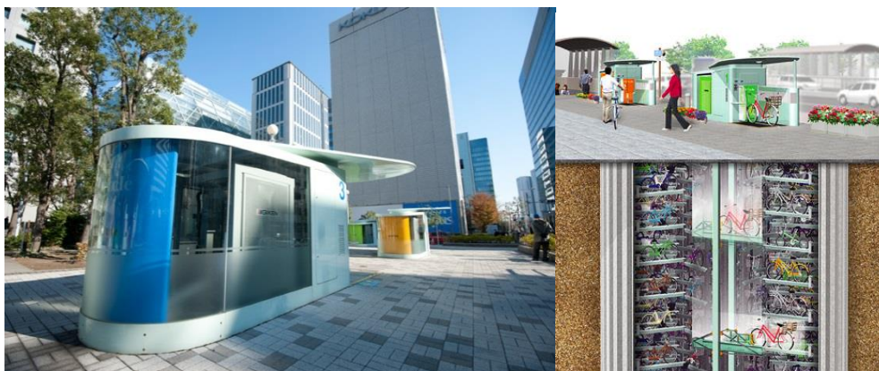
Plate 6.3 – Automated Cycle Storage (this shows an underground system)
