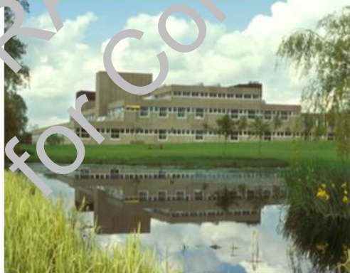
Cavendish II - View West across the pond
