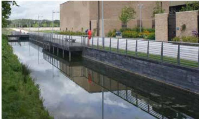
The canal is part of the site wide drainage system and is located between the Lake and Southern Residences. It is not linked to the pond in front of Broers building or the pond in the south east corner. Currently the water flow in the canal and the pond is not optimal and there are opportunities to connect them into a joint system and improve the flows and health of the canal.
