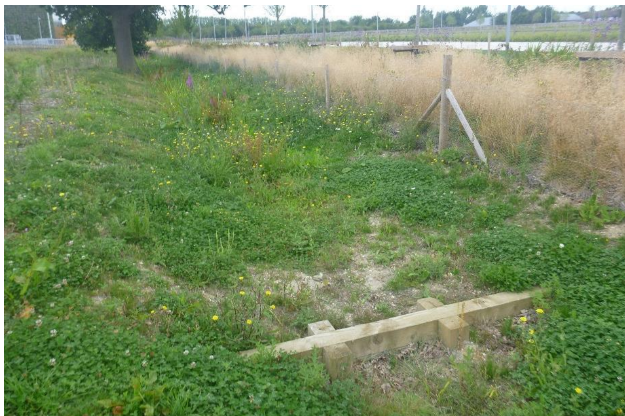
Figure 13.2 Channel looking upstream, with landscape planting (on true left bank), mature tree (on tree right bank) and low head weir structure in foreground
