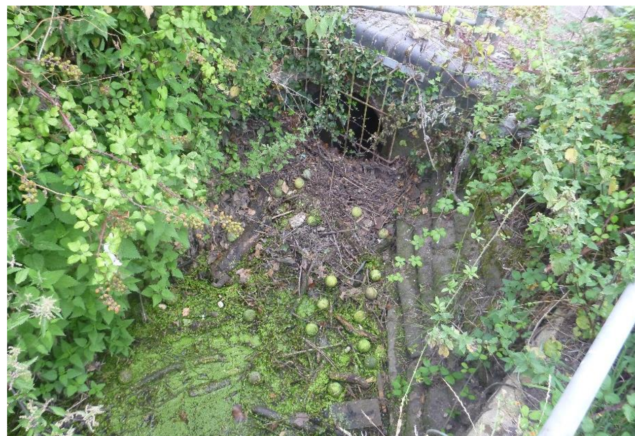
Figure 13.8 Culvert at Cambridge Lawn Tennis Club
