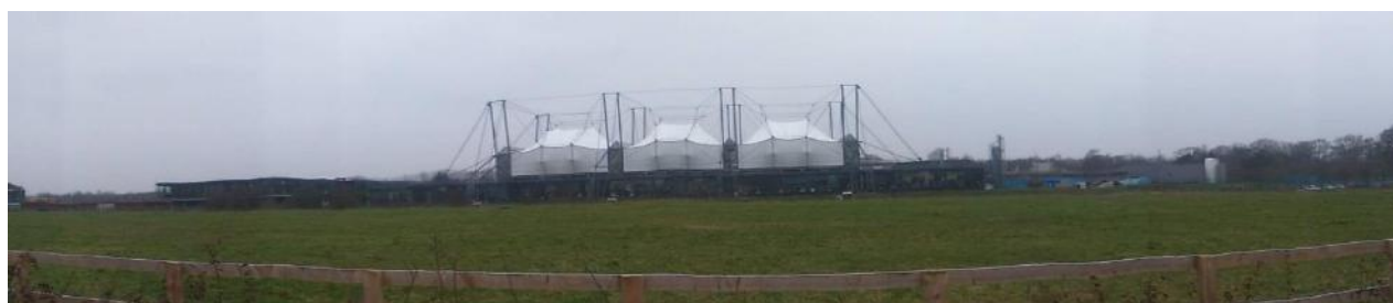
View 16 of the Schlumberger building
