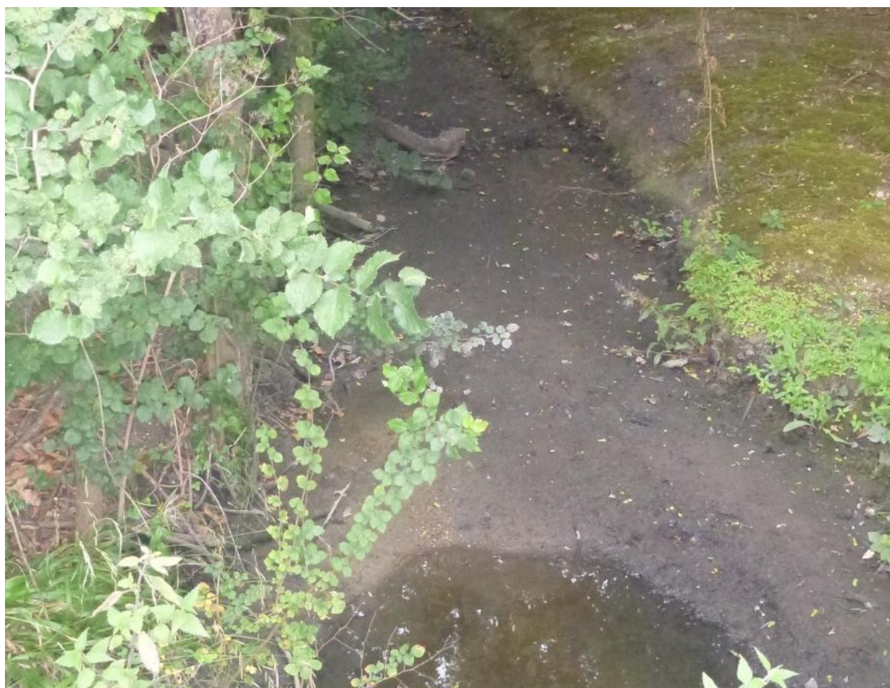
Figure 13.10 Immediately downstream of the A1303 looking downstream to silt accumulation
