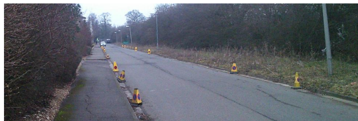
View 5 along Western Access Road / Ada Lovelace Road looking north
