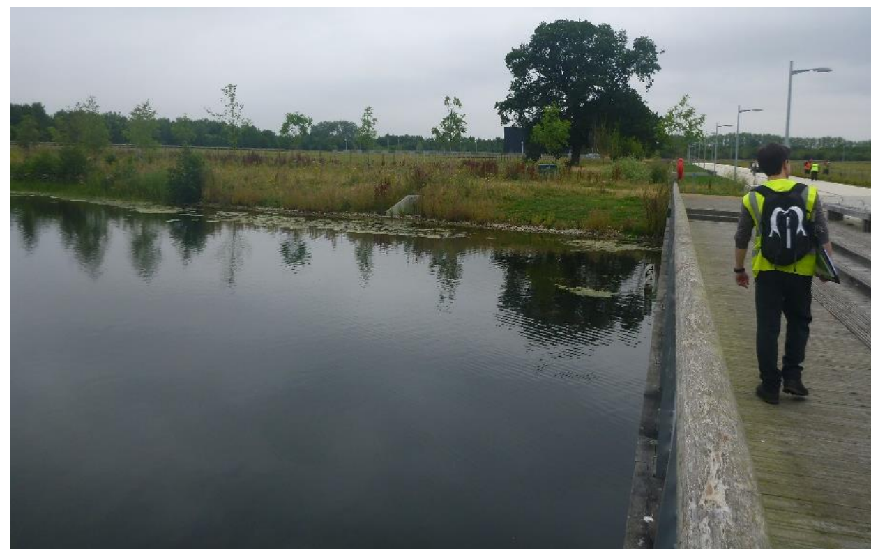
Figure 13.3 Looking upstream to outfall structure from Reach 1 into West Cambridge Lake, with landscaped platform on northern bank and soft landscaped western bank.
