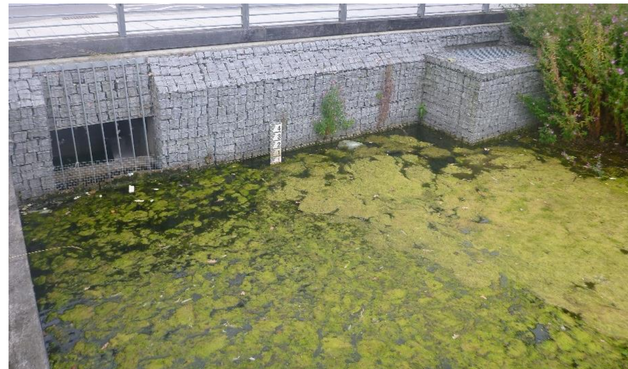
Figure 13.5 Outfall structures at downstream end of West Cambridge Canal with filamentous algae obvious on the water surface
