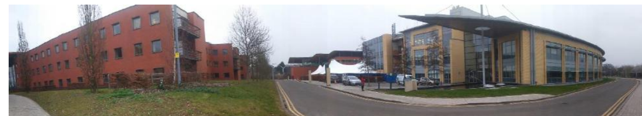
View 10 of the William Gates Building and the Centre for Advanced Photonics and Electronics
