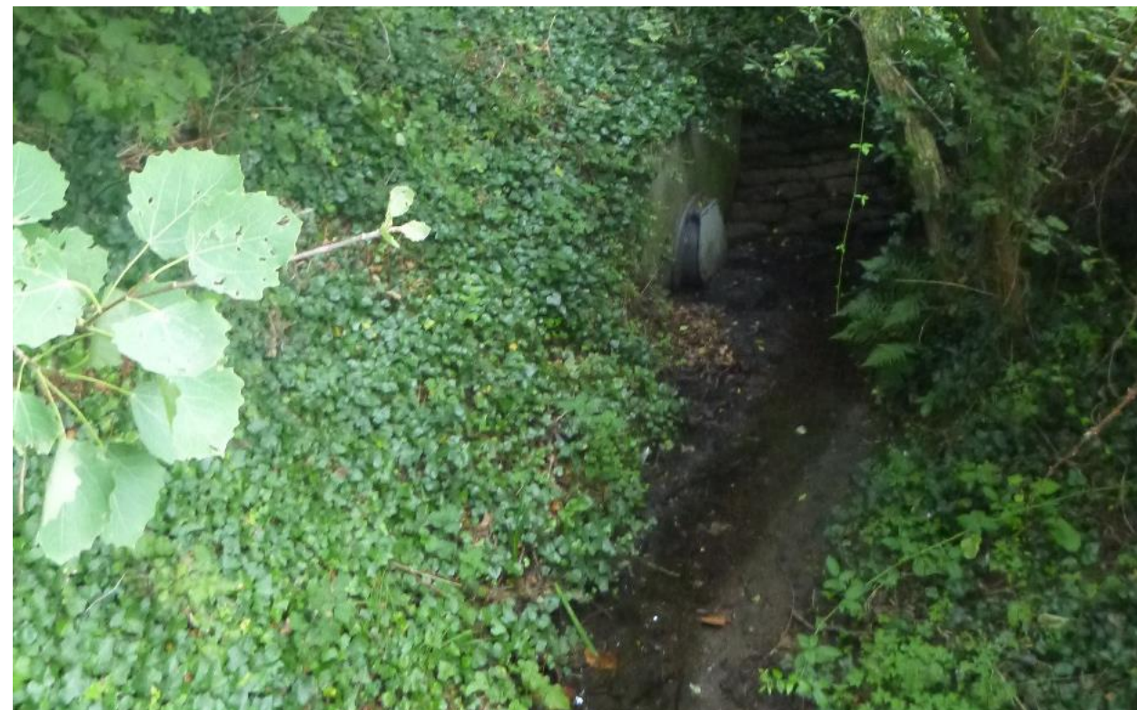
Figure 13.7 Flapped outfall with silt accumulation in heavily shaded channel
