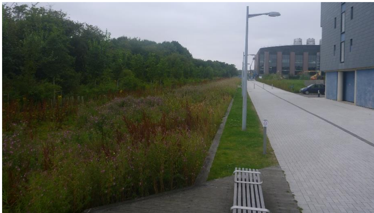
Figure 13.6 Swales, looking upstream within constrained corridor with vegetation masking the engineered structural diversity
