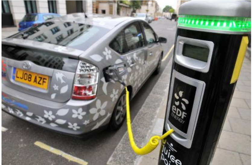
Electric charging points at different location, including car park buildings and internal garages will be planned (image: Charging Points).
