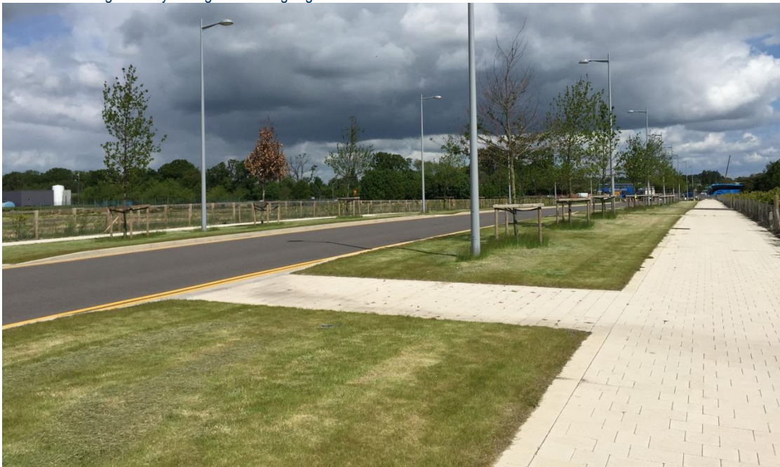
Plate 3 1: Existing Footway arrangement along High Cross
