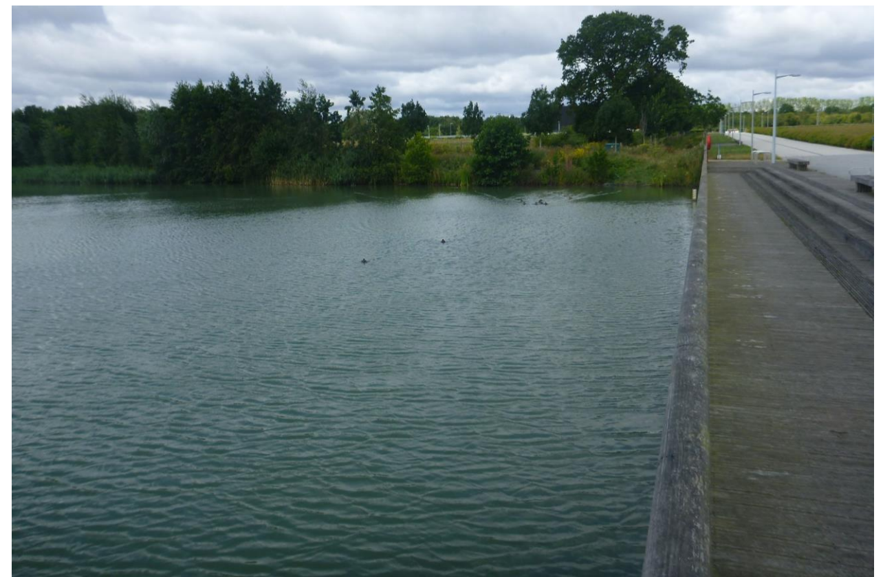
Figure 9.2 Looking upstream to outfall structure from Reach 1 into West Cambridge Lake, with landscaped platform on northern bank and established riparian vegetation along the western bank
