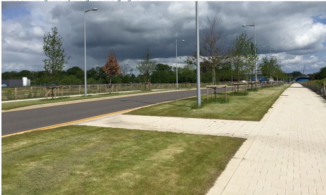
Plate 3.6: Existing Footway arrangement along High Cross
